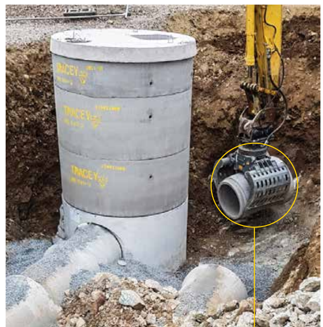
Rocker Pipe being installed
