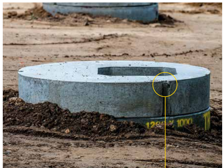
Cast in lifting loop
