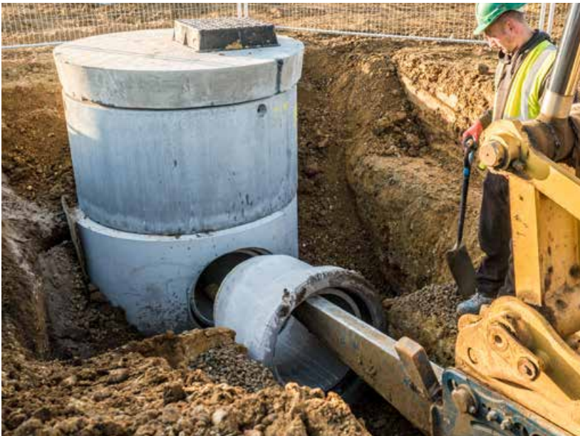
Rocker Pipe being connected to a Perfect Base™
