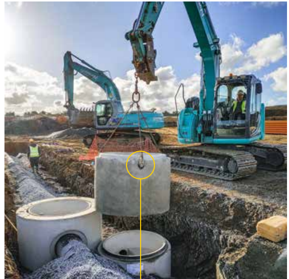
Lifting shackle mid lift
