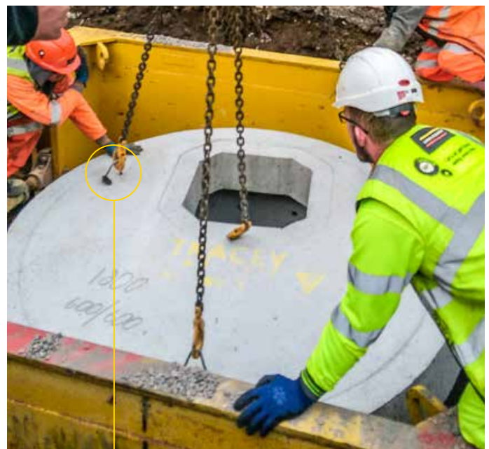
Cast in lifting loops
