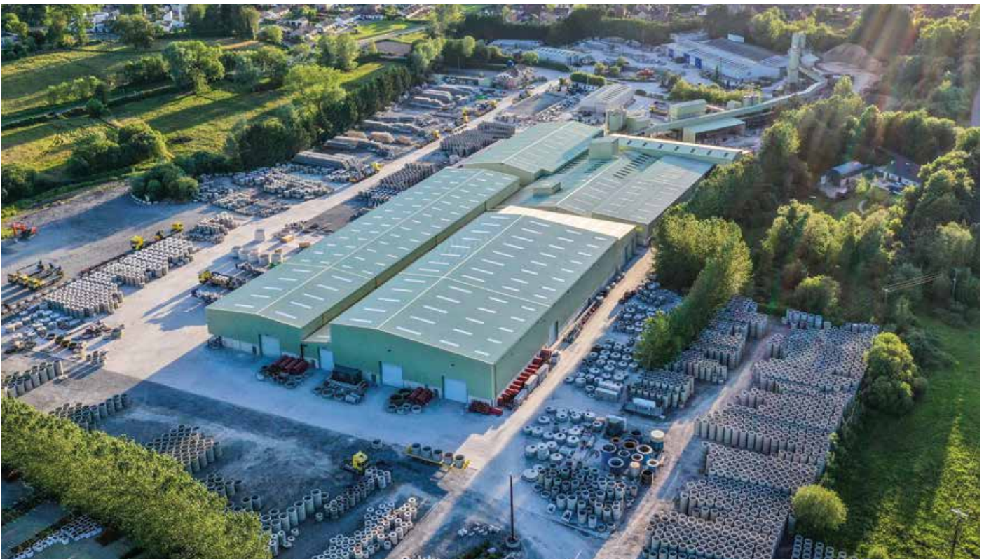
Tracey Concrete's Precast Drainage Factory - Enniskillen
